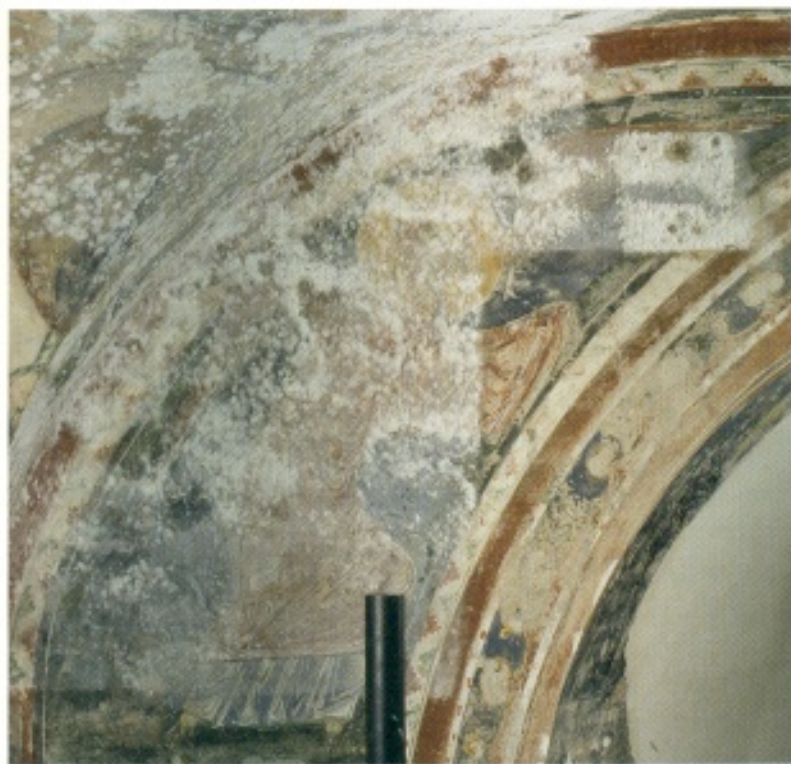
[19] Anagni Cathedral, Crypt. Microbiological infestation of fungi on the paint layer
