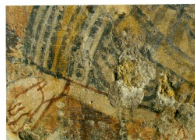
[3] Church of the Original Sin, Matera. Carbonate efflorescence around the edges of the fills added during restoration.
