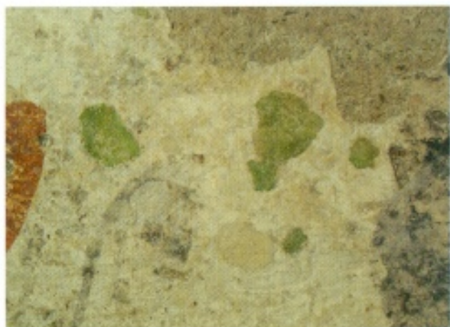
[5] Church of the Original Sin, Matera. The fills added during restoration have stimulated growth of green microorganisms.
