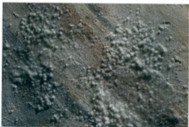
[9] Sanctuary of the Madonna, Paganica. A detail showing fungi growing on the paint layer.
