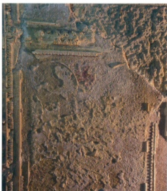
[14] Domus Aurea, Rome. Raked light, showing salts and the detachment and cupping of the thin, painted intonachino layer.
