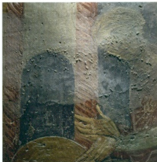
[18] Anagni Cathedral, Crypt. Salt efflorescence, fortunately limited and flaking paint
