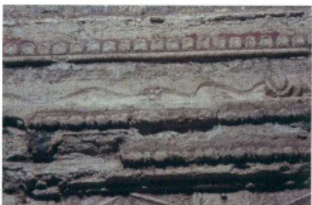
[15] Domus Aurea, Rome. Detail showing losses and powdering in the stucco decoration.
