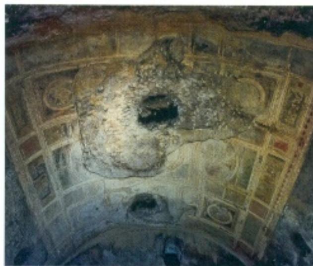
[12] Domus Aurea, Rome. General view of the vault before treatment. The white areas are sulphate incrustations of up to 5 mm in thickness.
