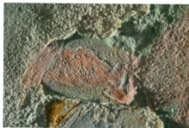
[8] Sanctuary of the Madonna, Paganica. A detail showing the severe powdering of plaster. The surviving paint layer here is so totally impregnated with synthetic resins that it has been completely denatured.
