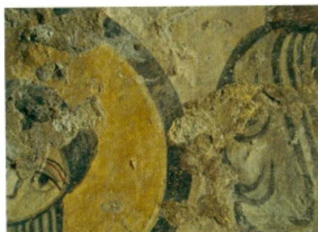
[2] Church of the Original Sin, Matera. Carbonate efflorescence around the edges of the fills added during restoration.
