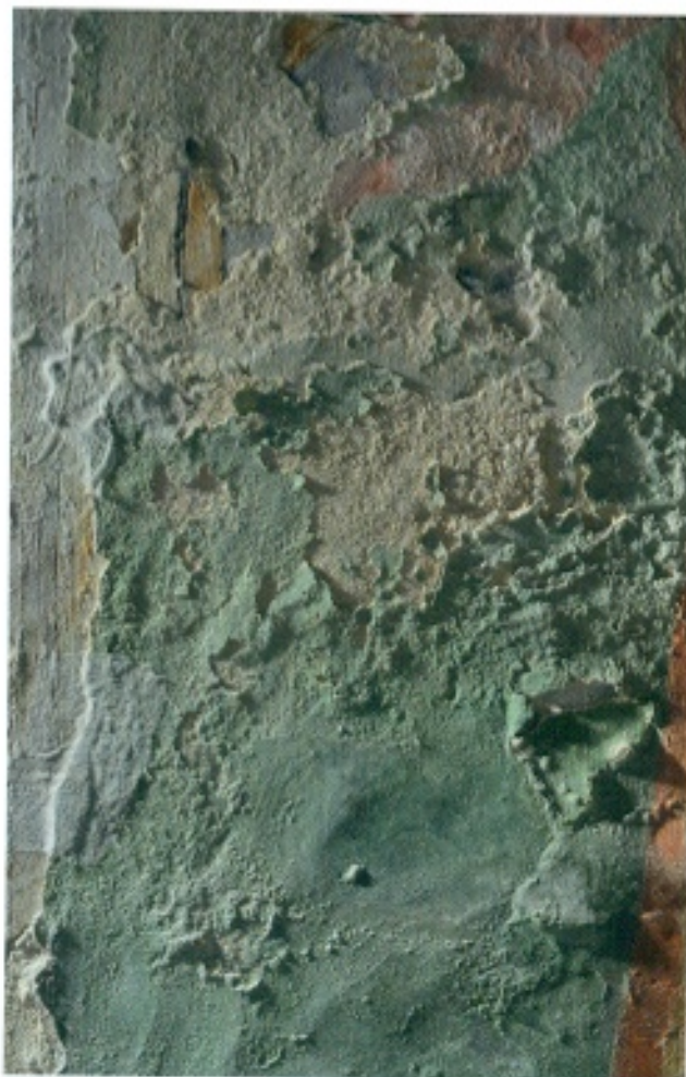
[7] Sanctuary of the Madonna, Paganica. Severe powdering of plaster and detachment of paint film. The paint layer here is heavily contaminated with synthetic resin.
