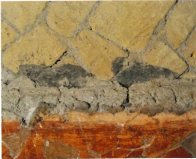
FIGURE 2.30. Coarse-grained mortar edging partially covering both anchoring mortar and backing plaster.
