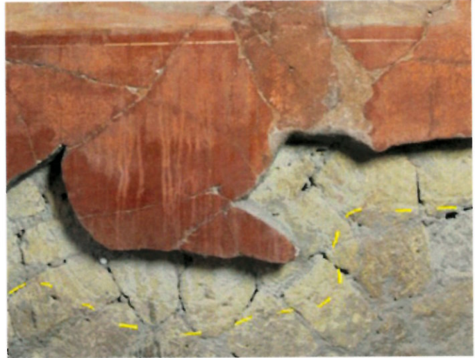
FIGURE 2.31. Lower edge, west wall. The lighter-colored strip (outlined by the yellow dashed line) is the location of the first sloped edging plaster.
