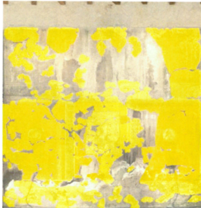
FIGURE 2.5. East wall. Yellow shading indicates original Roman plasters.
