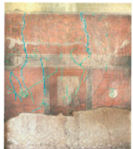
FIGURE 2.11. West wall. The yellow outline indicates an area without significant fractures. The thicker blue lines indicate cracks. The thin lines indicate fragments.
