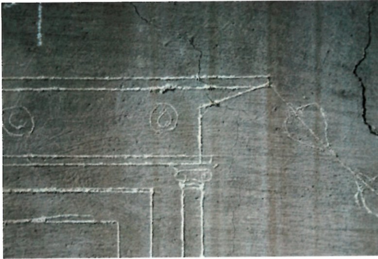
FIGURE 2.25. Reconstruction of the basic design of architectural elements on the upper east wall by Maiuri's team in area of large loss made by incising a line through a gray lime wash applied to the surface to reveal the thinly applied fine white lime plaster below.
