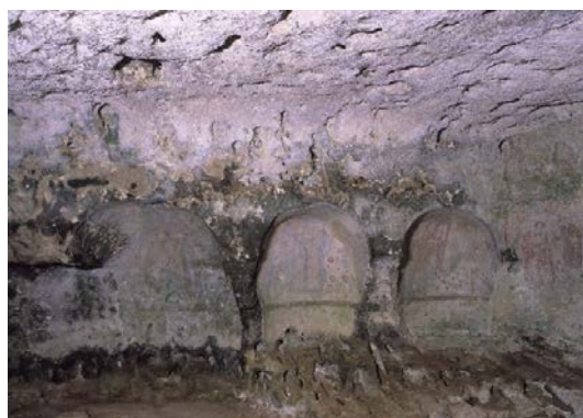
Fig.1a, b Wall A and B in 2003, before treatment
